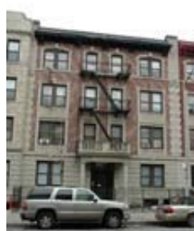
1150 President Street is a four-story, walk-up apartment building located in Brooklyn, New York City.
